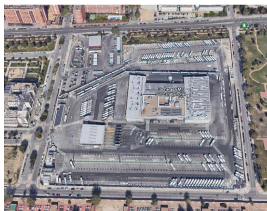
Figure 112: Madrid Mega site: Carabanchel EMT depot aerial image 3 .
